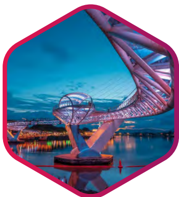
Darul Hana Bridge
