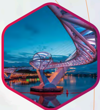
Darul Hana Bridge
